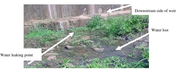
Figure 4: Leakage on Geray River Diversion
