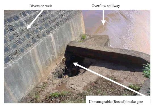
Figure 6: An intake gate of Fetam Diversion
