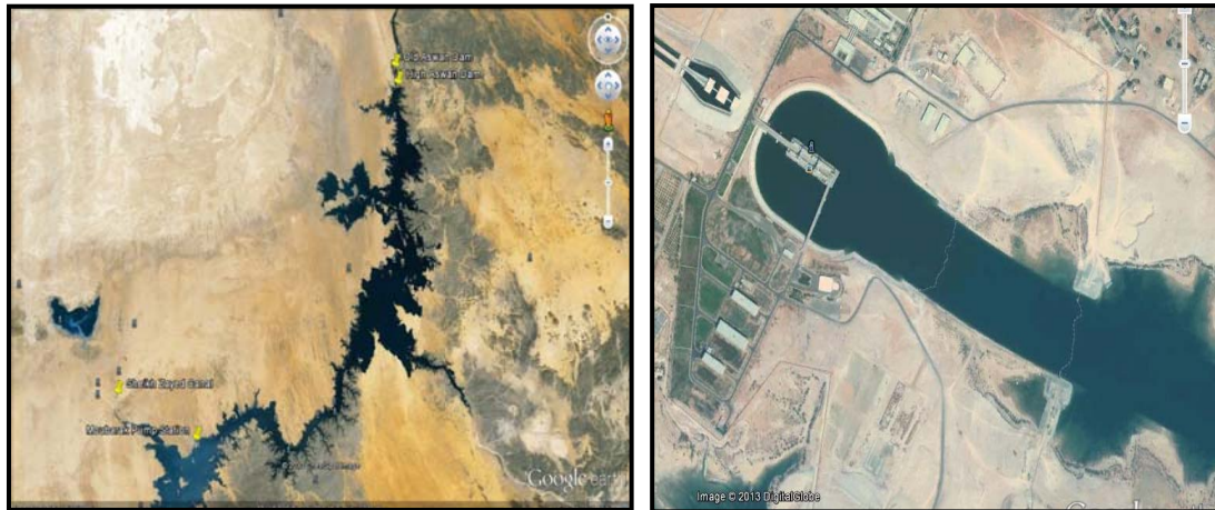
Figure 1: Satellite images show the location of Mubarak pump station on the western bank of Nasser Lake
